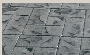
Stamped coloured concrete
