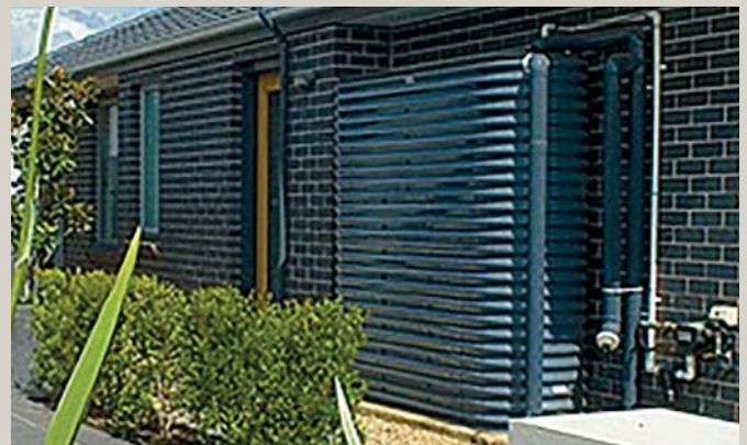
Slimline water tanks Integrated within the side setback of the building
