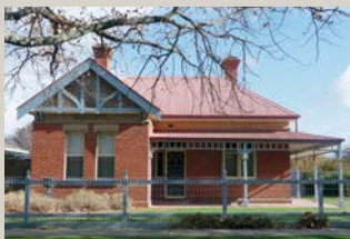
Gable facing the street, verandah an attached structure below roof line
