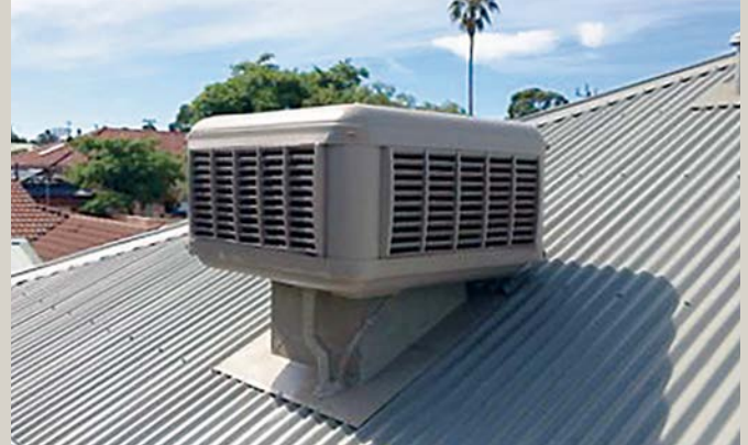
Low profile Evaporative Cooling Units mounted under the roof ridge line
