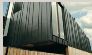
Metal sheet cladding
