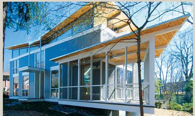
High quality architectural designs that respond to the site and the context
