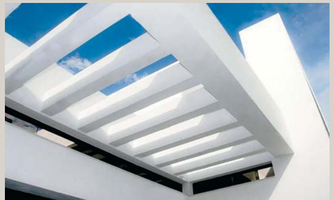
Shade structures and pergolas over garages and articulating front facades
