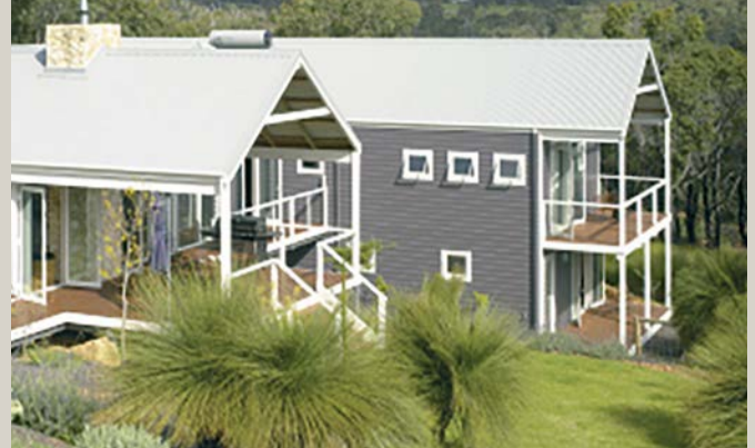
Accessible useable balconies on the upper levels
