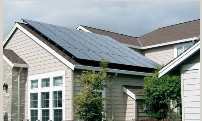
Solar panels integrated to roof design to reduce visual impact
