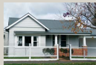
Woven wire fence with painted timber structure
