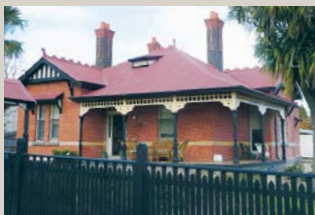
Verandahs wrapping the corner of buildings
