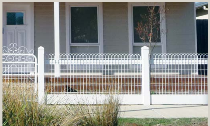
Woven wire front fence with painted timber work
