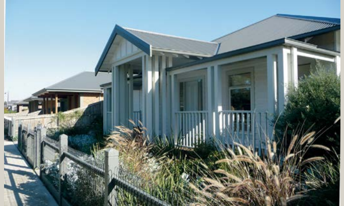
Woven wire front fence with boundary landscaping
