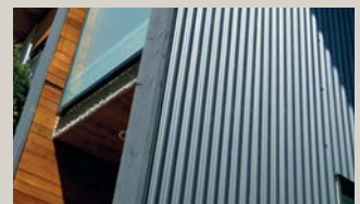
Vertical Colorbond cladding
