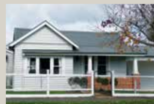
Woven wire fence with painted timber structure
