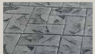
Stamped coloured concrete
