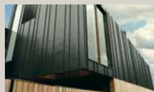
Metal sheet cladding
