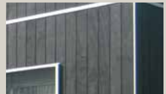
Vertical panel cladding
