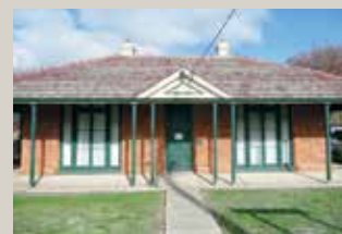
Brick veneer with slim line tiled roof
