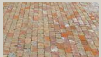
Brick and block pavers
