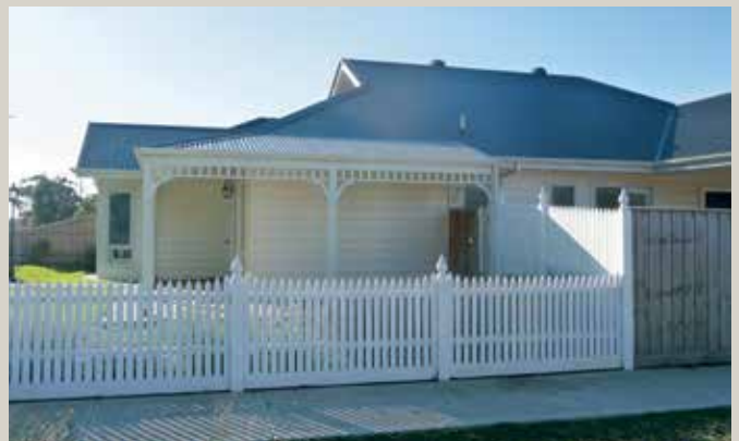
Front fence meets 1.8m side fence with no height taper
