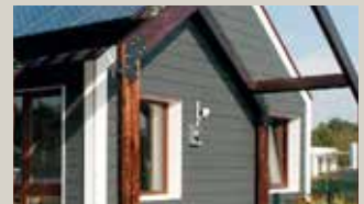
Horizontal panel cladding
