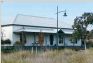
Elevated front verandah creating vertical separation encouraging use of the verandah
