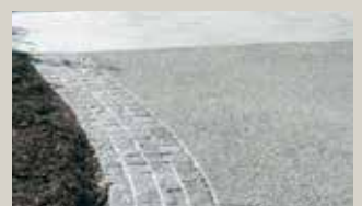
Mixed finishes & defined edges
